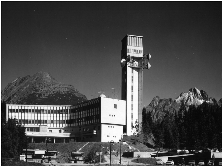
Štrbské Pleso: Communications building , from 1969-1970, Oľga Ondrejčíková
